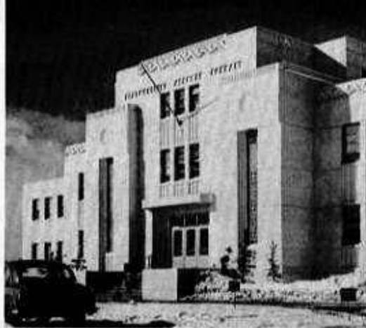
This modern building at Elmendorf AFB houses headquarters of the Alaskan Air Command.
