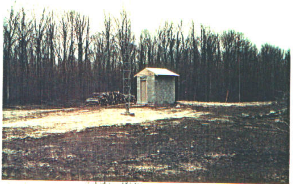
USDA Forest Service radio tower and auxillary building.
