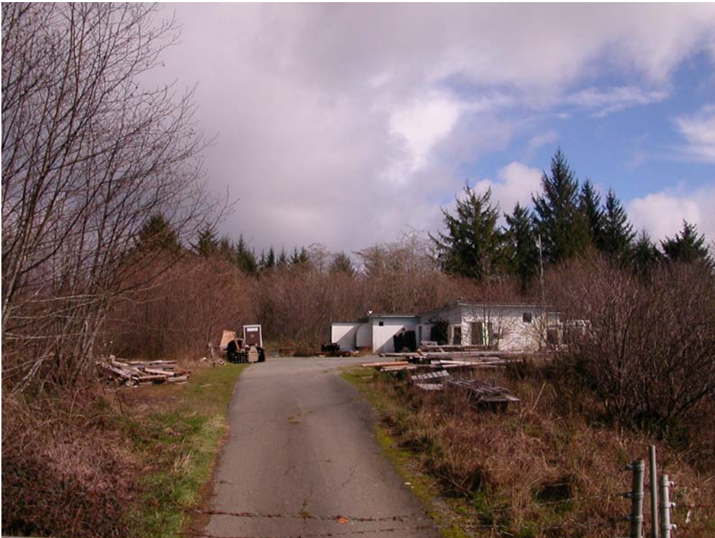
Figure 18 The GATR facility; note site debris
