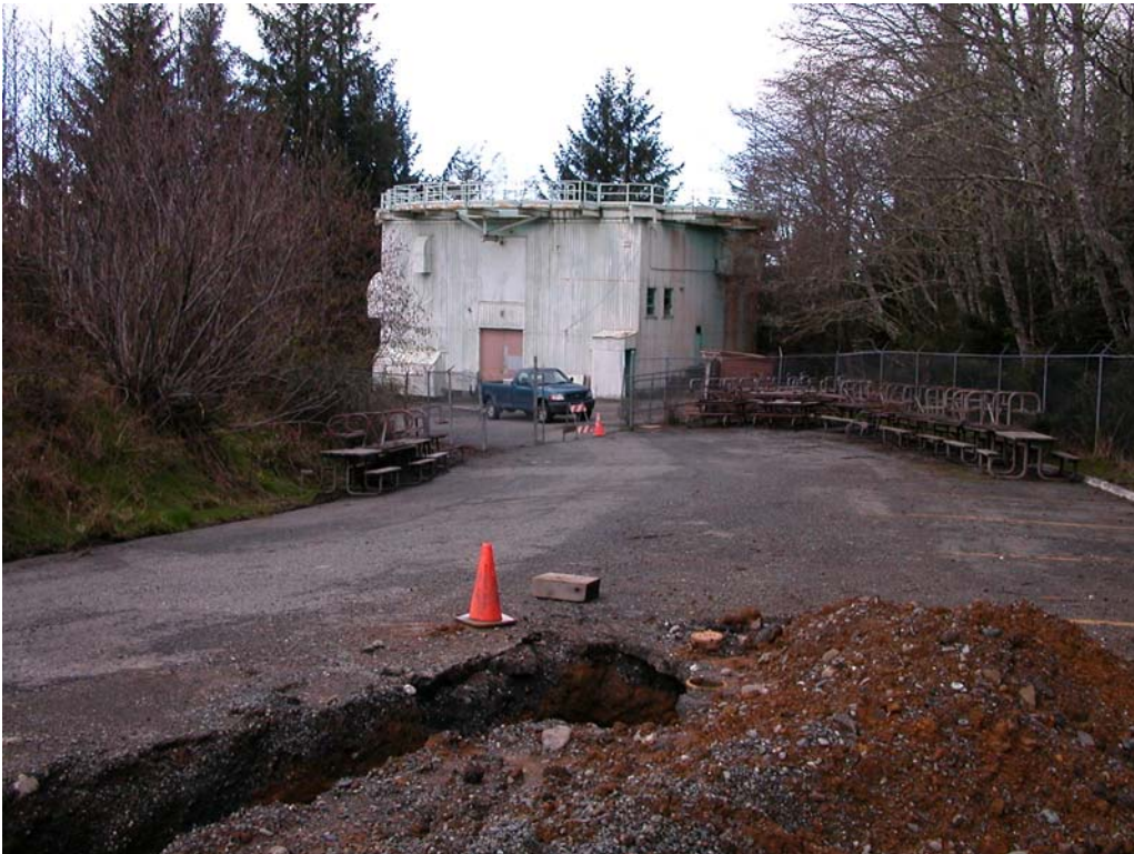
Figure 4 Building 98, with the Radome removed.
