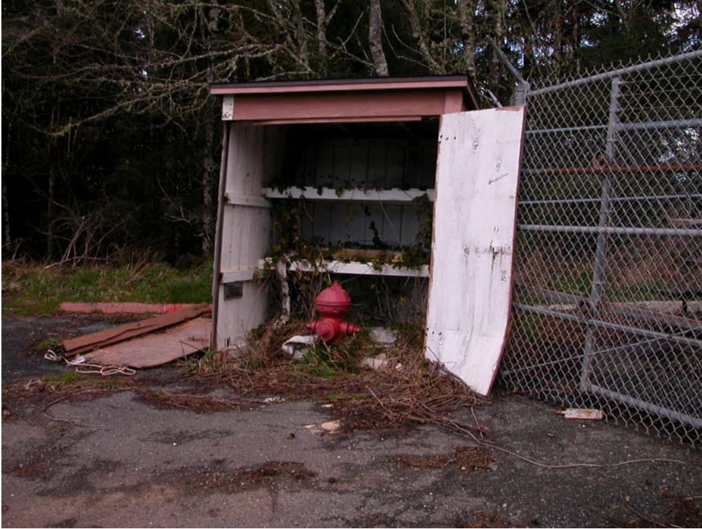
Figure 5 One of the many Fire Hose Houses throughout the RAFS
