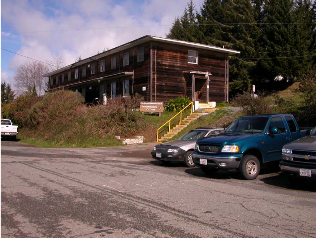
Figure 13 Building 200, now the National Park Offices
