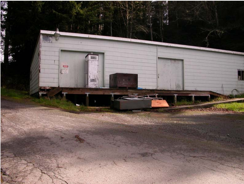
Figure 8 Building 109, closed due to asbestos contamination
