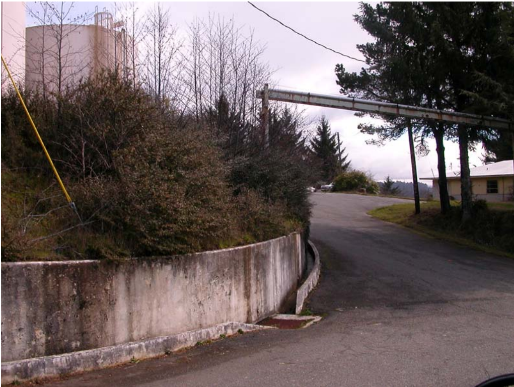
Figure 6 The water towers (Buildings 1024 and 1025), as well as the remains of the trestled water system which used to crisscross the property
