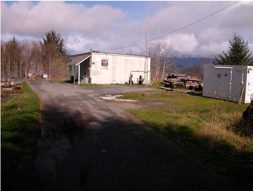
Figure 10 Building 150, the Ceramic Shop; note site debris surrounding building
