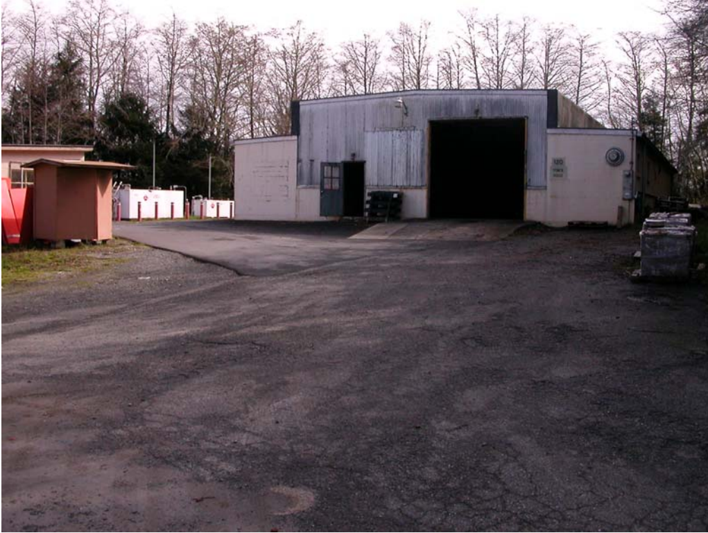
Figure 9 Building 120, the Power House; note ASTs in the background
