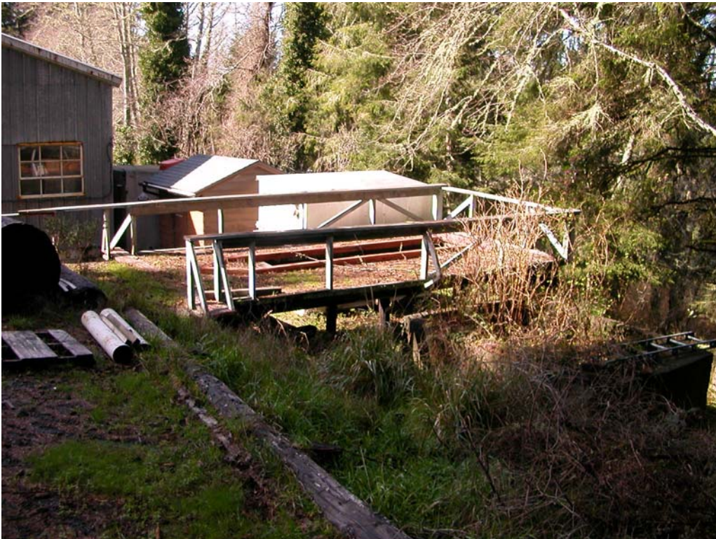
Figure 12 The Vehicle Maintenance ramp
