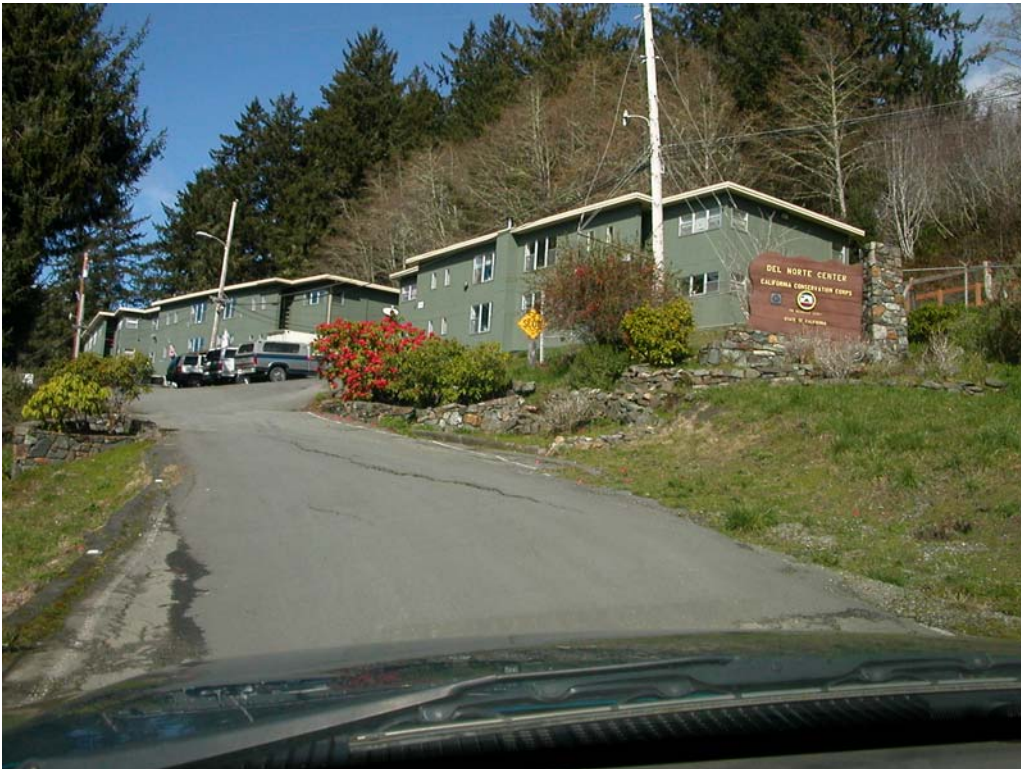
Figure 14 The CCCs facility, Building 300 in the foreground
