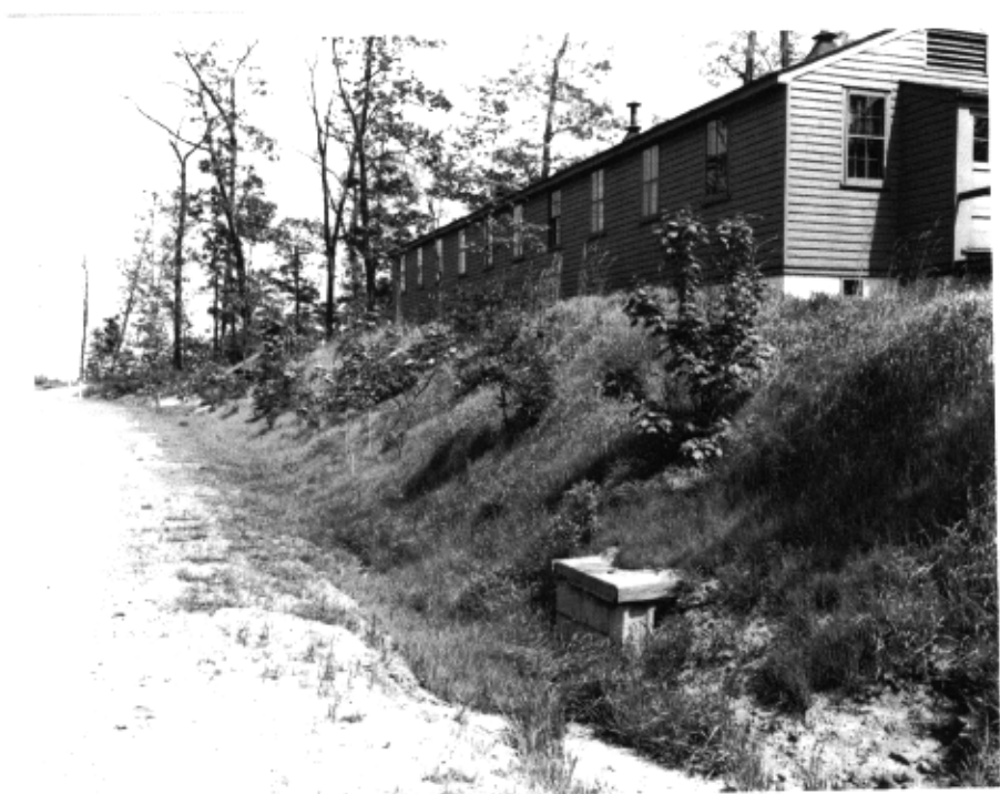
NJ_Monmouth County_Navesink Military Reservation_H62. Eastern Cantonment Barracks T-804 for 42 men, view south, c1944, GATE
