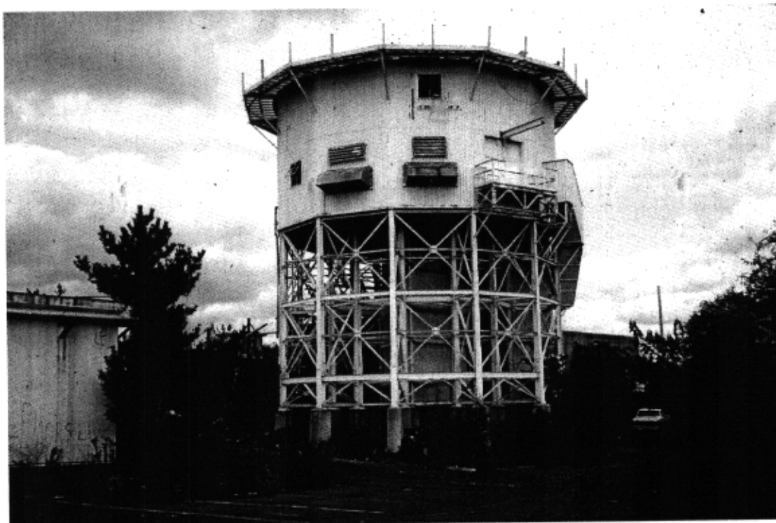
NJ_Monmouth County_Navesink Military Reservation_H88. Highlands Army Air Defense Site, Radar Tower, 1983, MCPS
