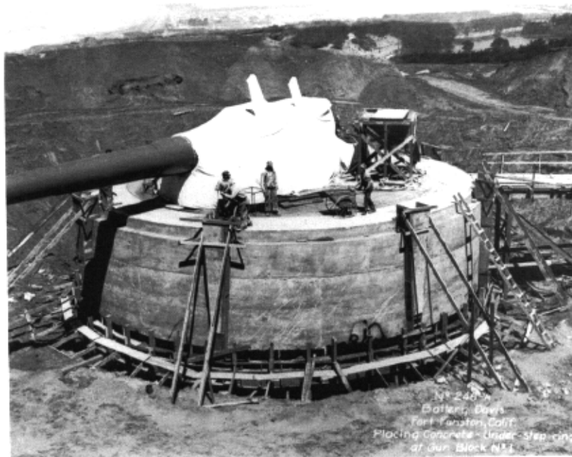
19. Gun block with 16-inch gun, Battery Richmond P. Davis, Fort Funston, HD of San Francisco. NARA Photo.
