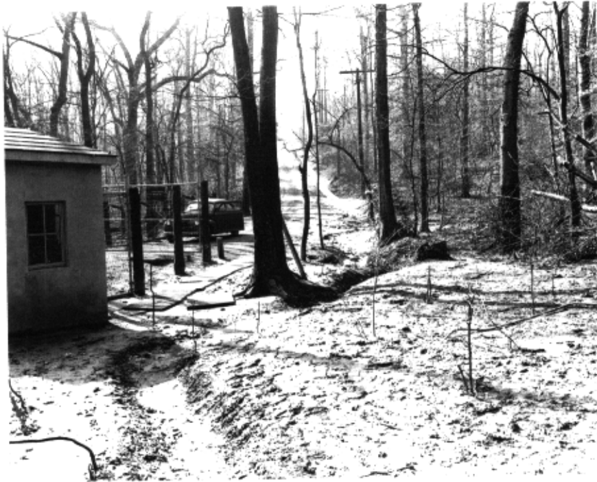
NJ_Monmouth County_Navesink Military Reservation_H63. Access Road E, Sentry Box and Gates, view south, c1944, GATE
