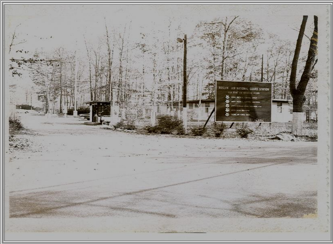
Main gate of the Roslyn ANG Station
