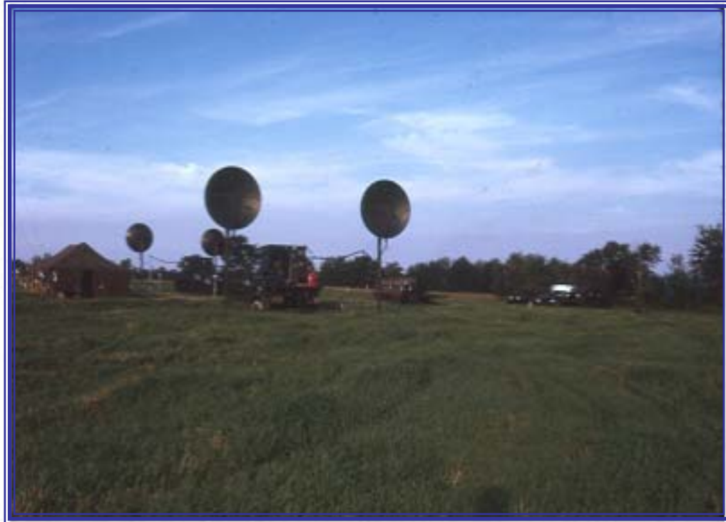
AN/TRC-97D Repeater Site showing 8 foot Parabolic dish Antennas
